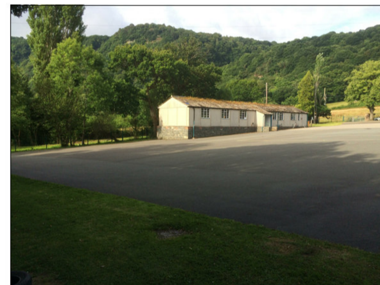
Image G - Existing Canteen Block
