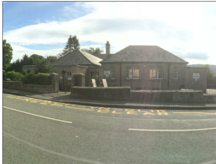
Image D - Existing Road Elevation
