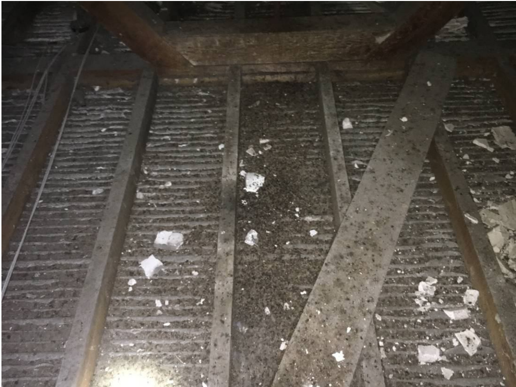
Significant quantities of bat droppings consistent with those produced by brown long-eared bats throughout roof voids 1, 2, 3 and 5.
