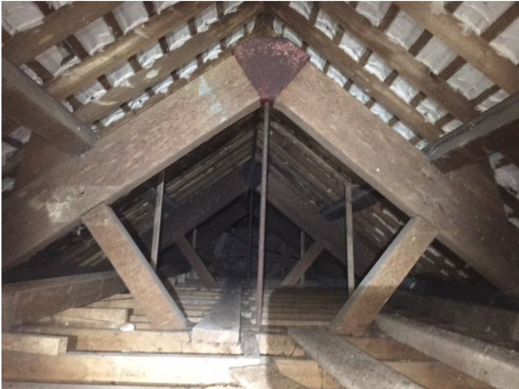
Internal view of roof void 5
