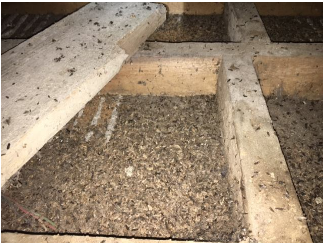
Significant quantities of bat droppings consistent with those produced by brown long-eared bats throughout roof void 5.
