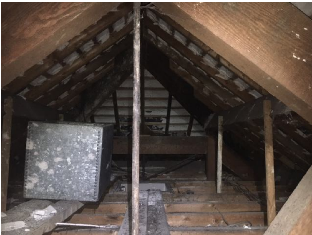
Internal view of roof void 4
