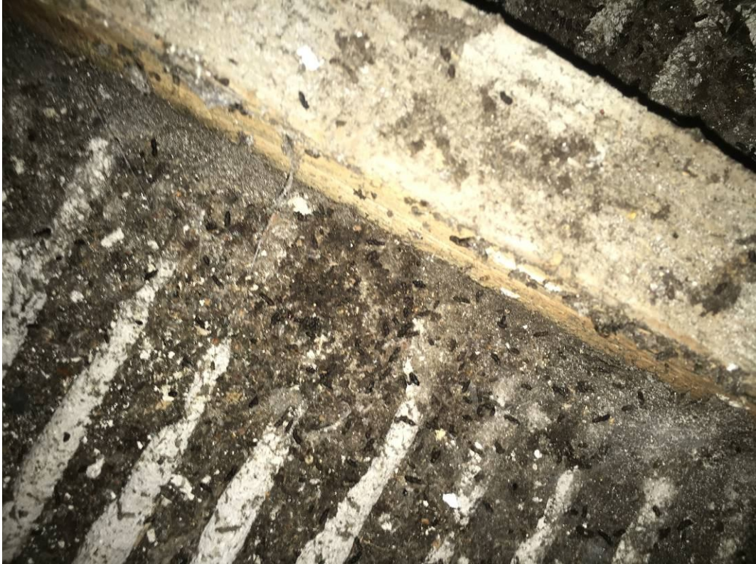
Small quantity of bat droppings consistent with those produced by pipistrelle or small Myotis bats within roof void 6.
