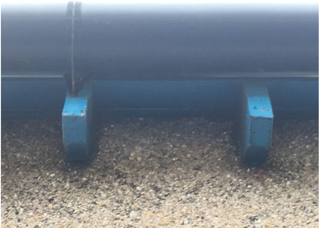
Well sealed wall tops, exposed rafter end roof design
