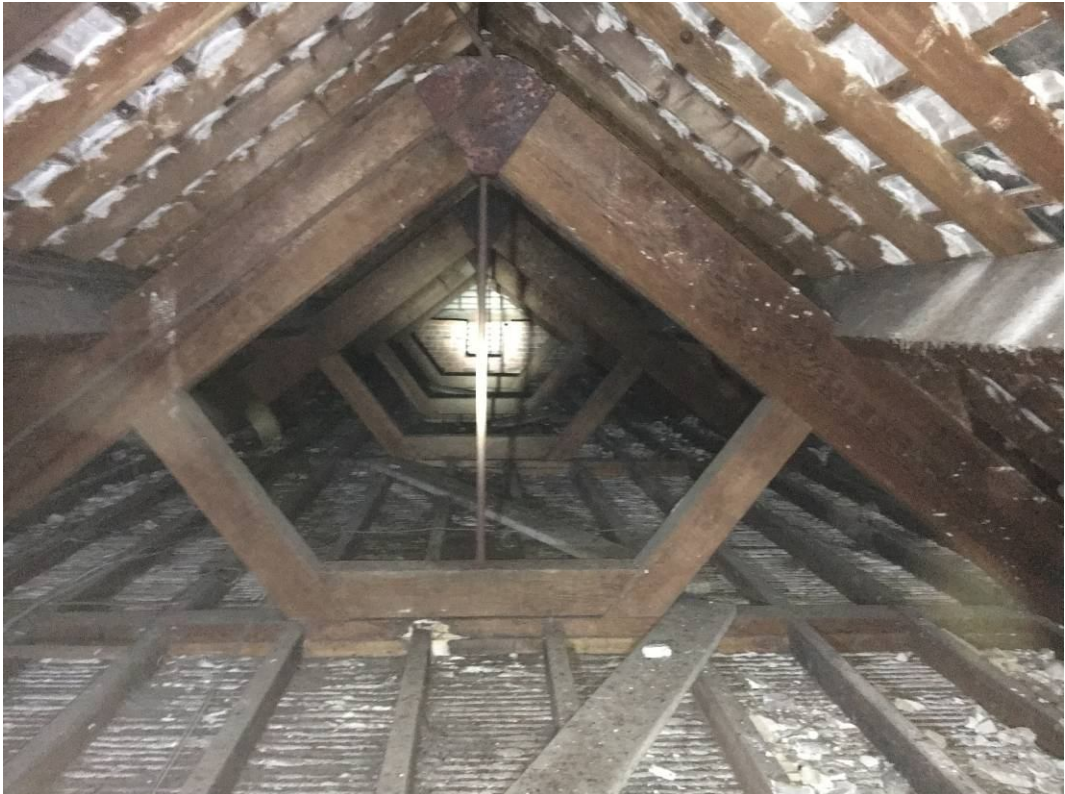
Internal view of roof void 1
