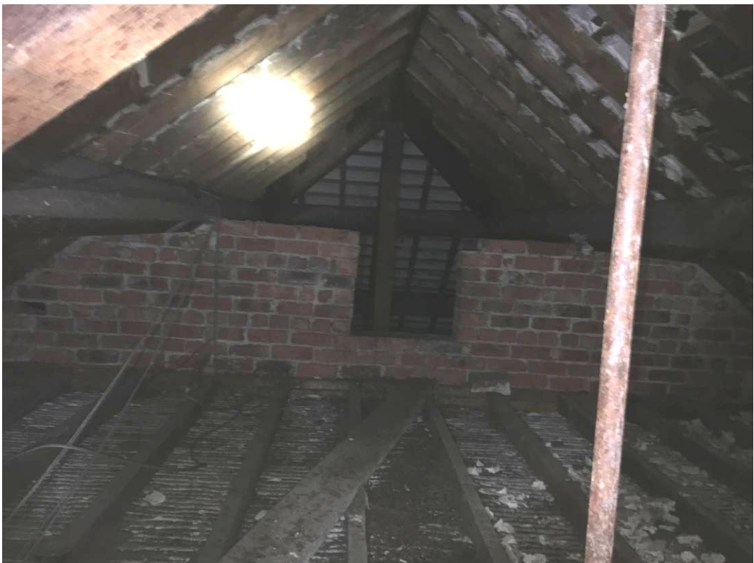
Internal view of roof void 1
