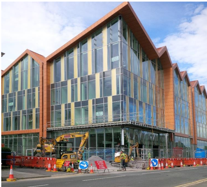
The external cladding now complete
