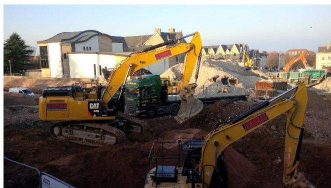
Construction Work on Site
