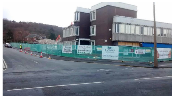
December 2016 - During demolition
