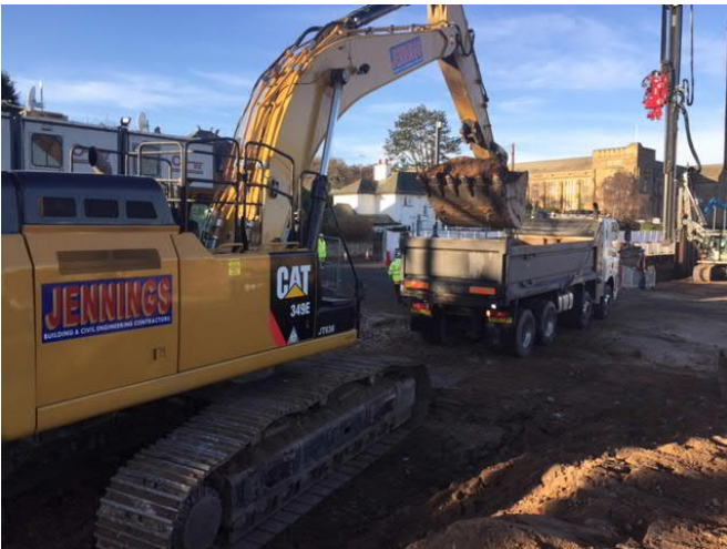
Jennings working on site
