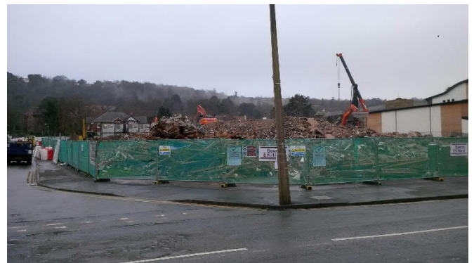
January 2017 - Demolition completed
