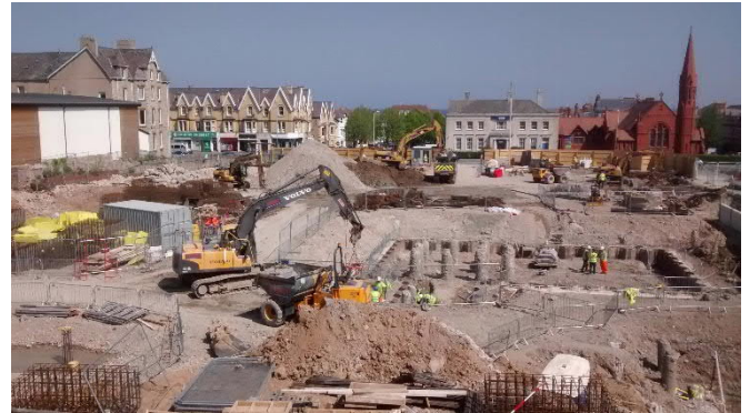
Pile capping, plant and machinery on site.
