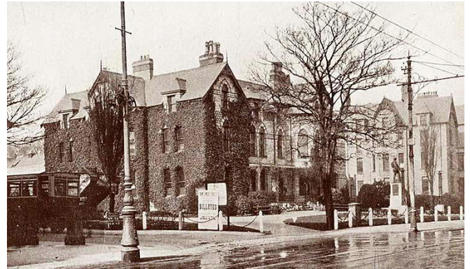
Old Town Hall, Coed Pella, Colwyn Bay (provided by The Colwyn Bay Heritage Group).
