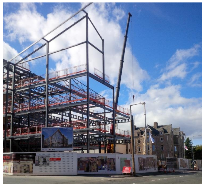
Above- work in progress, early October 2017
