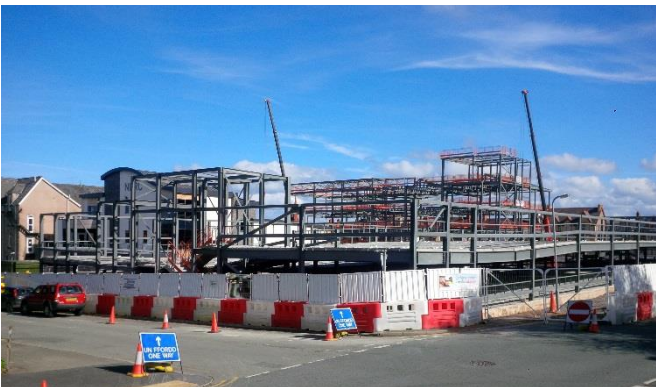
Above – car park in progress.
