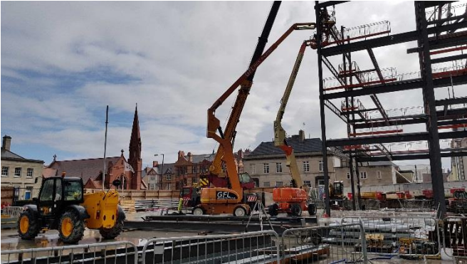
Above – early work on the office steel frame.
