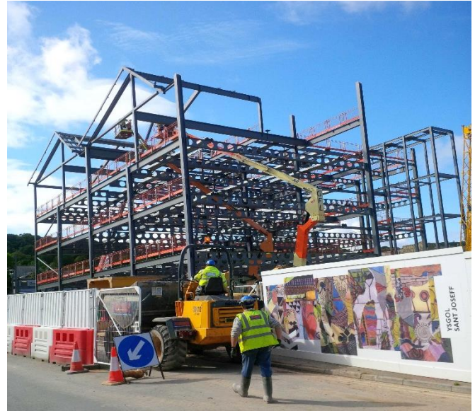
Above – office steel frame in progress.
