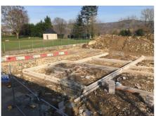
Demolition work on the old Ysgol Dolgarrog school has now been completed by K&C Construction, following their site occupation in November 2017. Following the demolition and general site clearance, the setting out and ground works have begun for the new Caerhun and Trefriw area school as well as the installation of the attenuation tank and the tanking of below ground walls.
