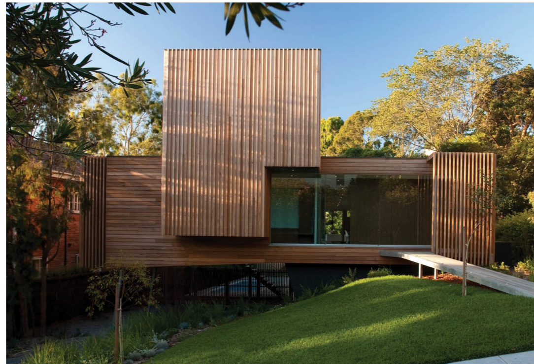
Sgrins pren a gwydr Timber cladding and glass
