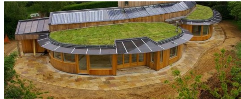
To gwyrdd (sedum) a solar Green (sedum) solar roof
