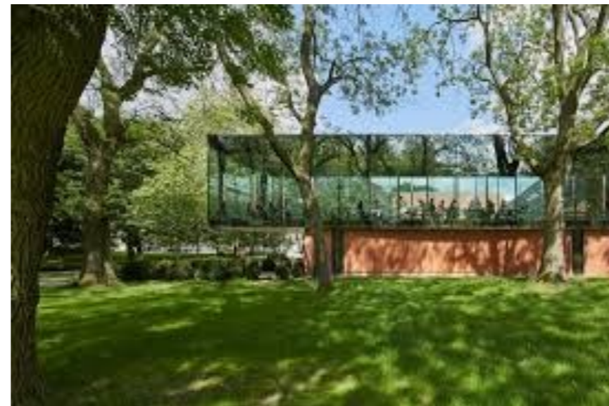
Pren a gwydr Timber cladding and glass
