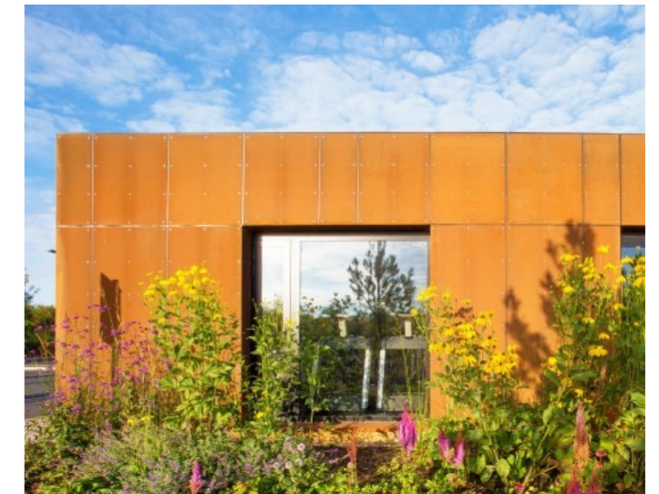
Sgrin law dur Cor-Ten Cor-Ten steel rainscreen cladding
