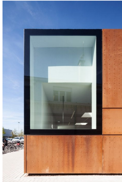
Sgrin law dur Cor-Ten Cor-Ten steel rainscreen cladding
