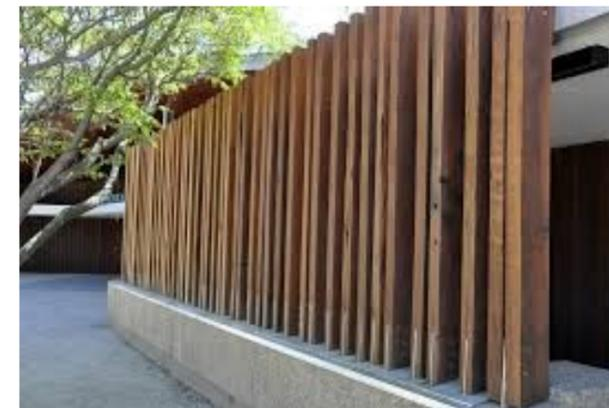
Use of timber : screening and general use in external works
