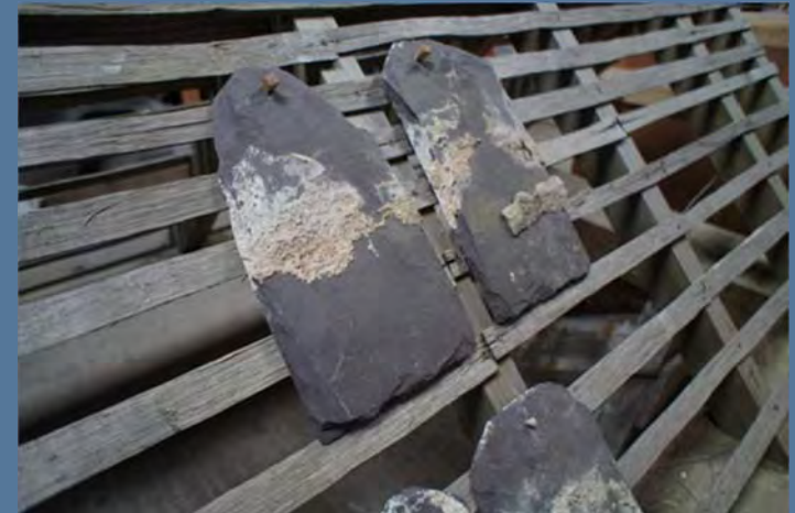
Above: Traditional pegged-slate roofing which lasts centuries and can easily be repaired.
