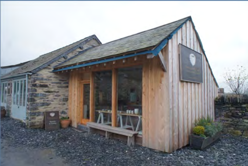
The Natural Building Centre, Llanrwst
