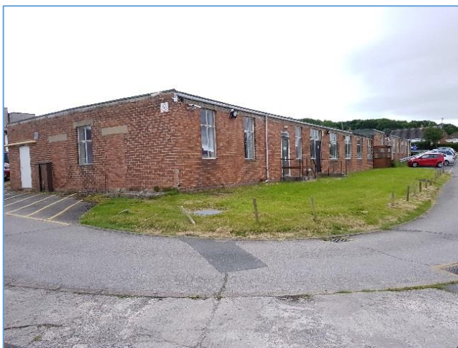
One of the many accommodation blocks at Dinerth Road.
