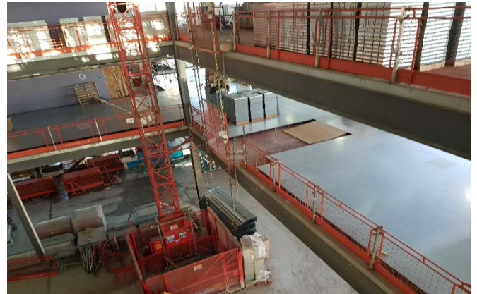
Above: Raised floors being laid on the upper levels.
