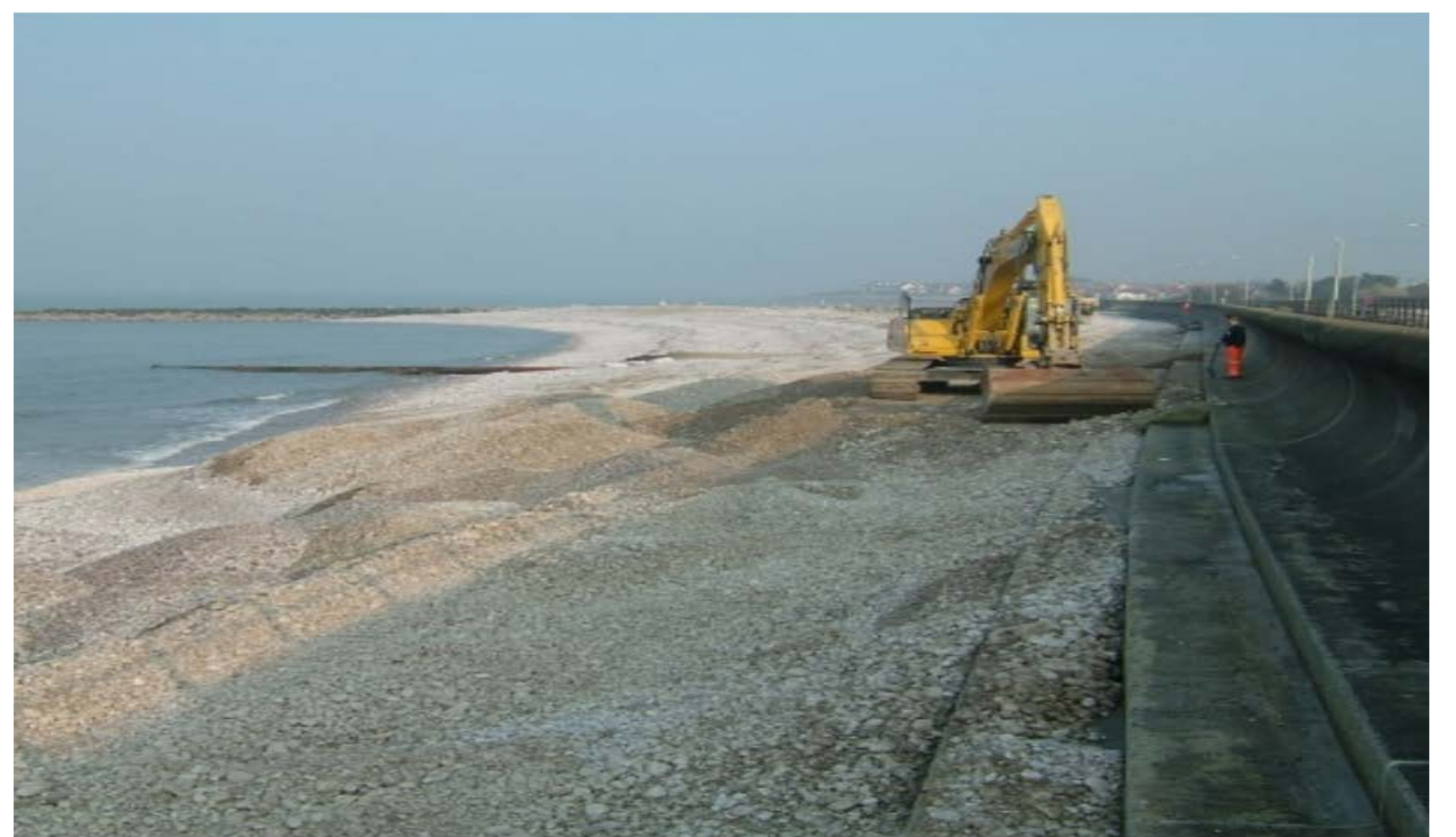
CCBC REGULARLY MOVE BEACH MATERIAL BACK TO THE CENTRE OF THE BAY AT SIGNIFICANT COST. THIS OPTION WOULD GREATLY REDUCE THE SPEED OF BEACH EROSION AND THEREFORE REDUCE THE FREQUENCY OF THIS TASK.
