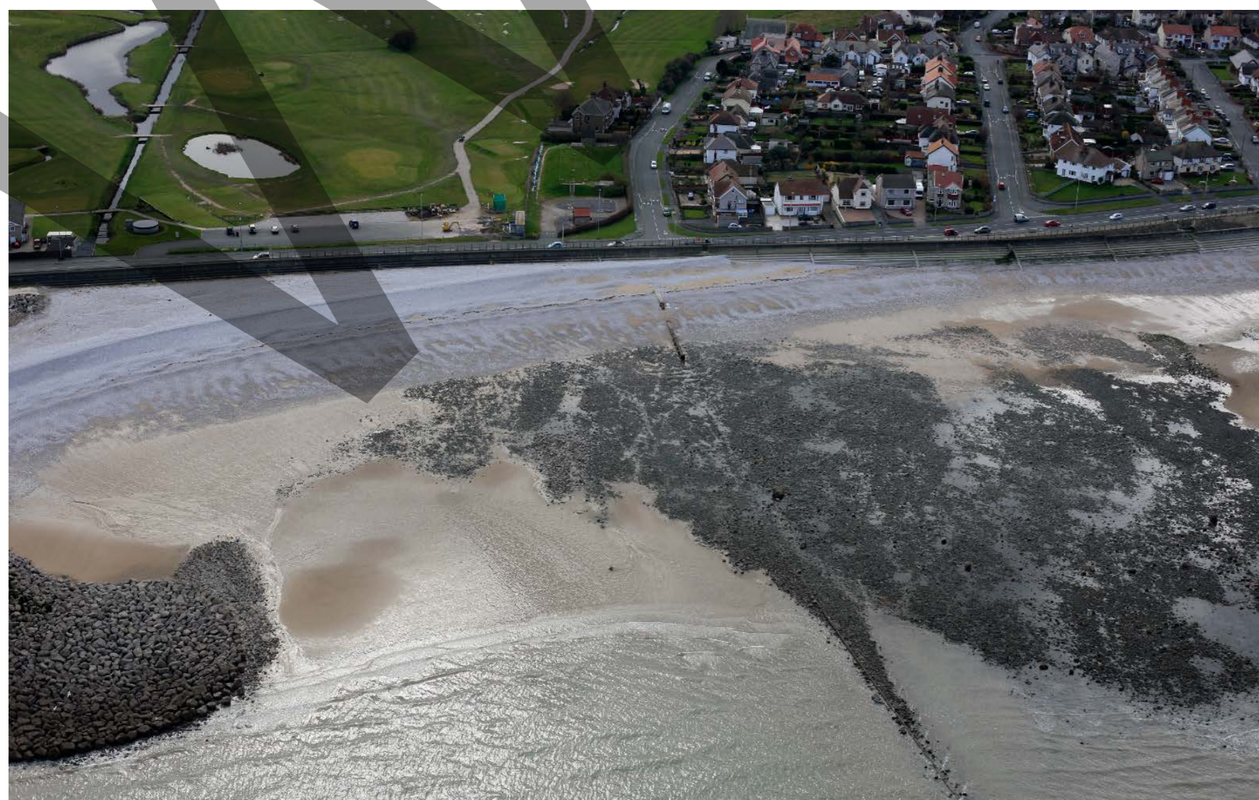
VIEW SHOWING THE SECTION OF THE BEACH THAT WE WOULD MODIFY AND RECHARGE WITH NEW MATERIAL UNDER THIS OPTION. THE EXISTING BREAKWATER CAN BE SEEN TO THE LEFT. THIS WOULD BE RAISED.
