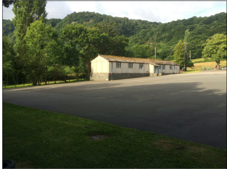
Image G - Existing Canteen Block
