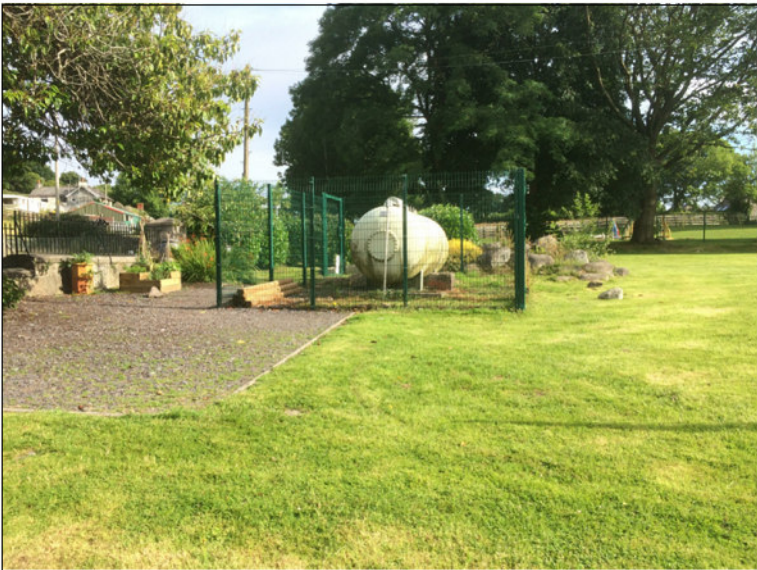
Image A - Existing Gas Tank
