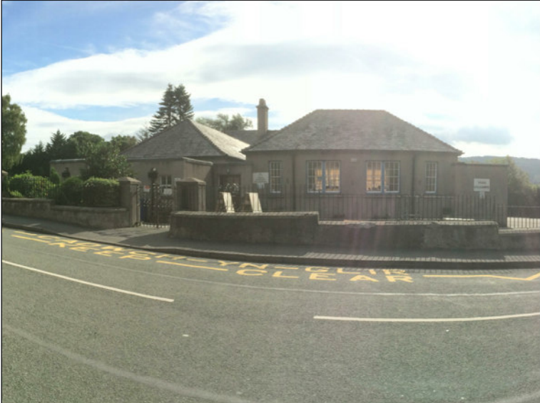
Image D - Existing Road Elevation
