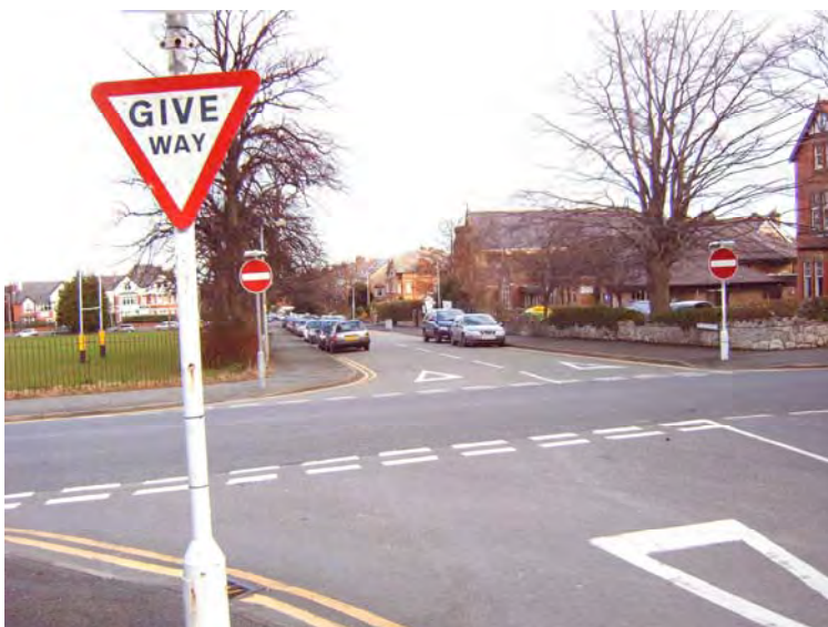
Street furniture and road markings
