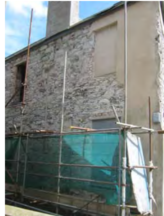
Renovation work on exterior walls
