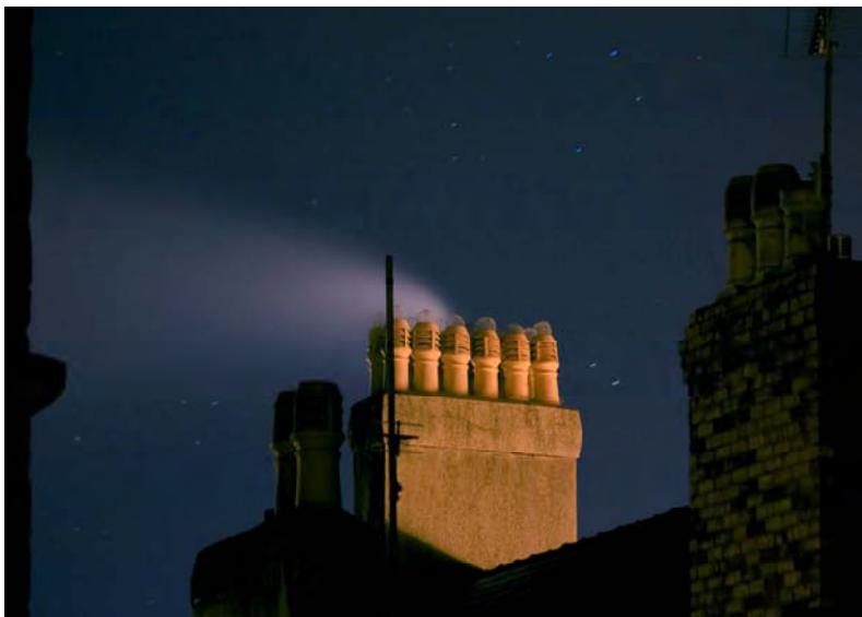
Chimneys add character to the appearance of a conservation area
