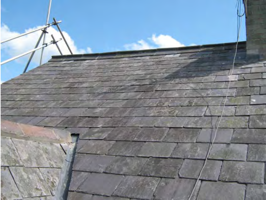
Example of a refurbished slate roof
