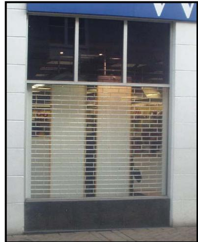
5.3 The size and location of grilles will be determined by the window opening. They may be retracted during opening hours into box housings, usually located within or behind the window soffit.
