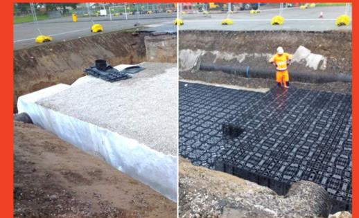
The lefthand image shows the crates covered with the geotextile and the protective layer prior to backfilling. The righthand image is during the crates being placed.
