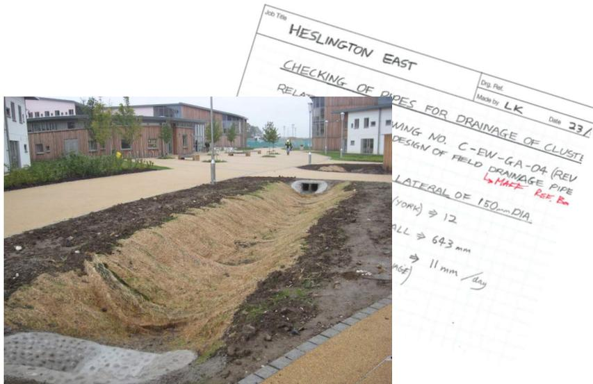
Swale immediately after construction showing the biodegradable erosion protection blanket, Heslington East campus, University of York, YO10 5DD
