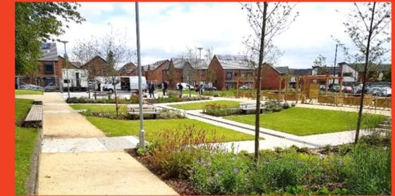
Paths and hard surfaces have been replaced by permeable paving, additional areas of highway storm water runoff are drained into infiltration ponds and rain gardens which are planted with biodiverse vegetation and allow residents to enjoy.
