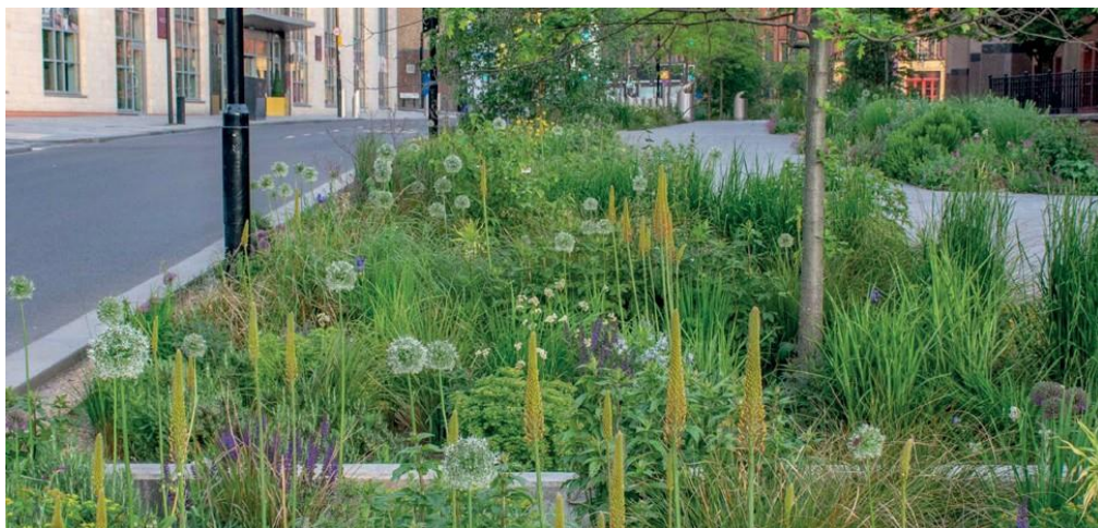
Sheffield Grey to Green rain garden planting providing SuDS to take stormwater runoff and enhancing biodiversity in the city centre Image Source: Nigel Dunnett
