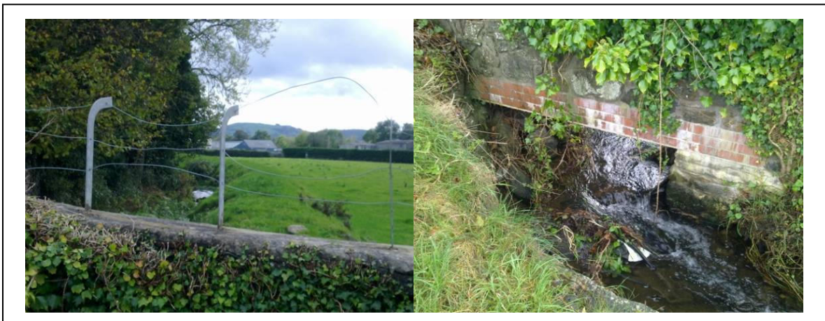
Figure 4.16 – Photos of Flood Bank and Opening through Wall
