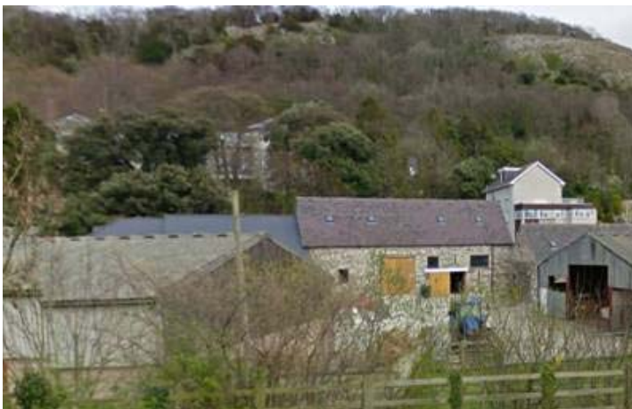
Figure 6 – Marl Farm, Marl Lane, Llandudno Junction. Conversion of outbuildings into four dwellings.
