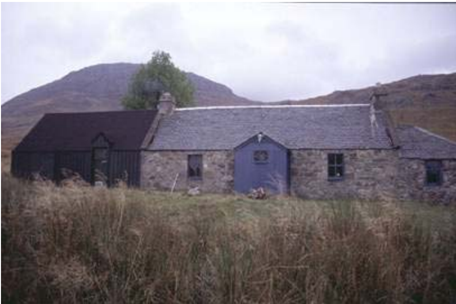
Figure 4 - Ben Alder Cottage in the Highlands - Example of an extension which was clad in corrugated black tin.
